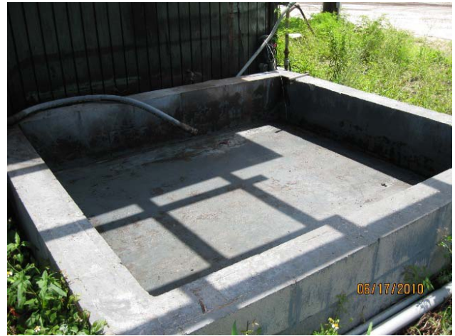
4. Secondary containment area at debarking-area shed after cleanup
